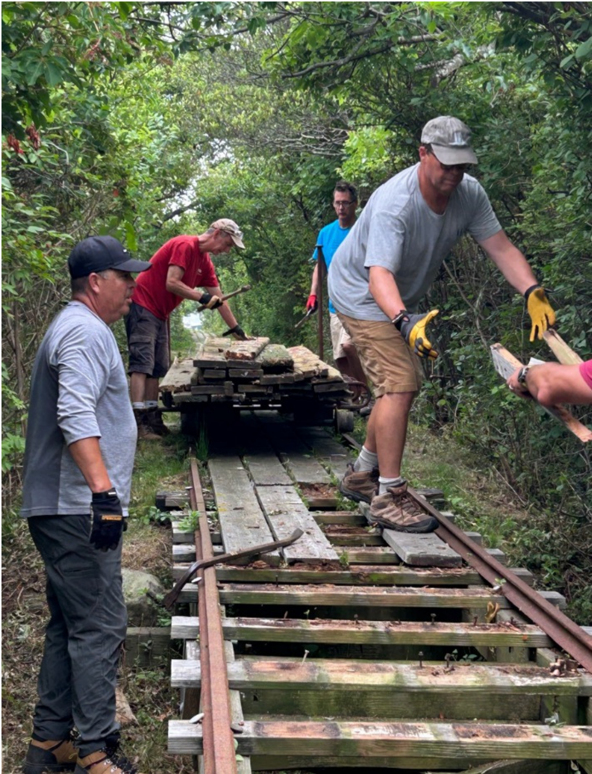
Volunteers Johnnie Martinez, David Kearns, Mike Hammerl, and David Narkewicz remove old wood in preparation for rebuilding the Thatcher Island tramway.
