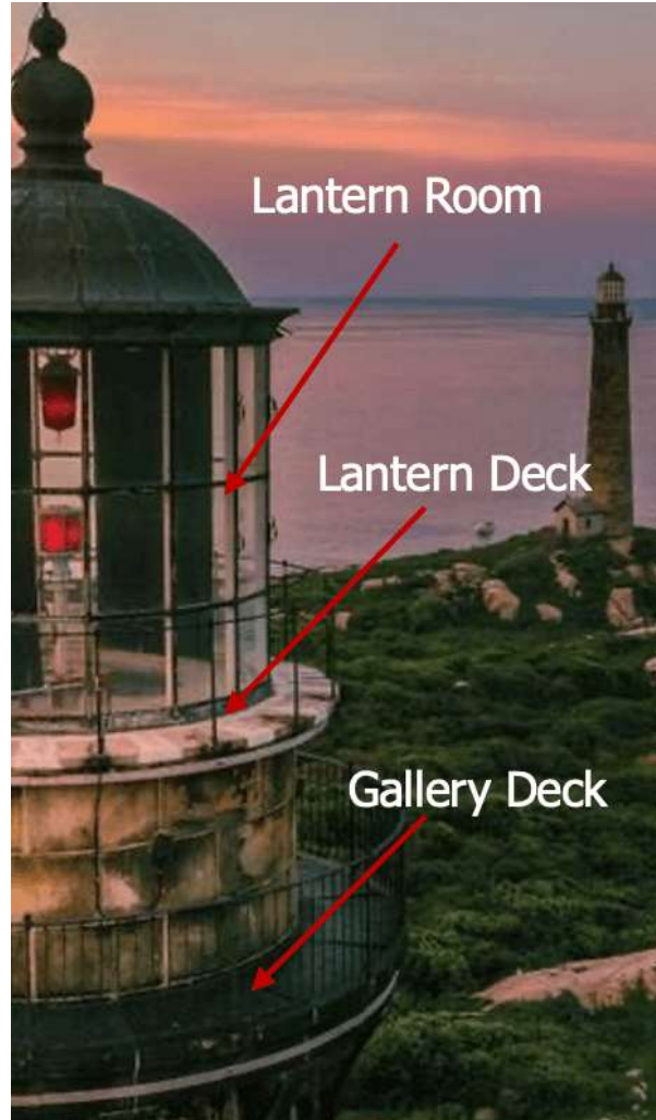
The South Tower Lantern Room, Lantern Deck, and Gallery Deck - the critical upper structures exposed to the full force of Atlantic weather. Image courtesy Thacher & Straitsmouth Islands Association.
