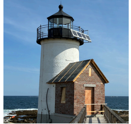
Partially completed Straitsmouth lighthouse entry cabin. Photo credit: Bill Whiting
