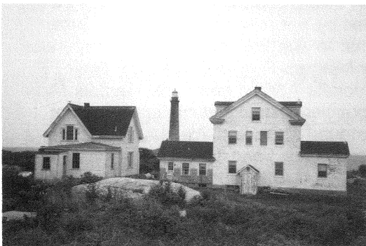
Principal keeper's house on left and Assistant keeper's house on the right from the back.
