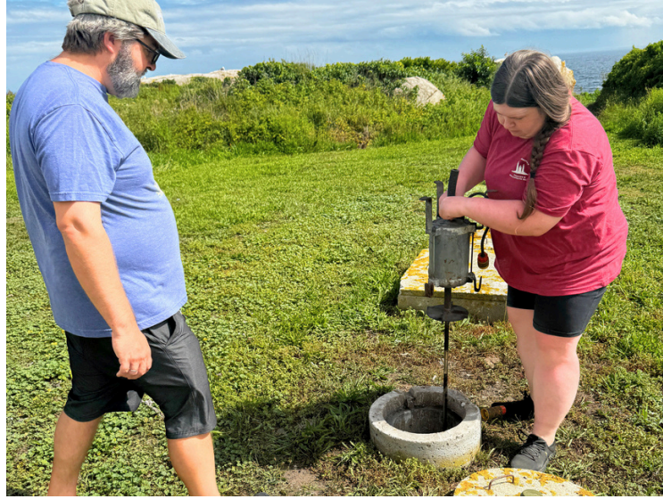
Nathan Cohen and Julianna Hul clean the sewage aerator on Thacher.
