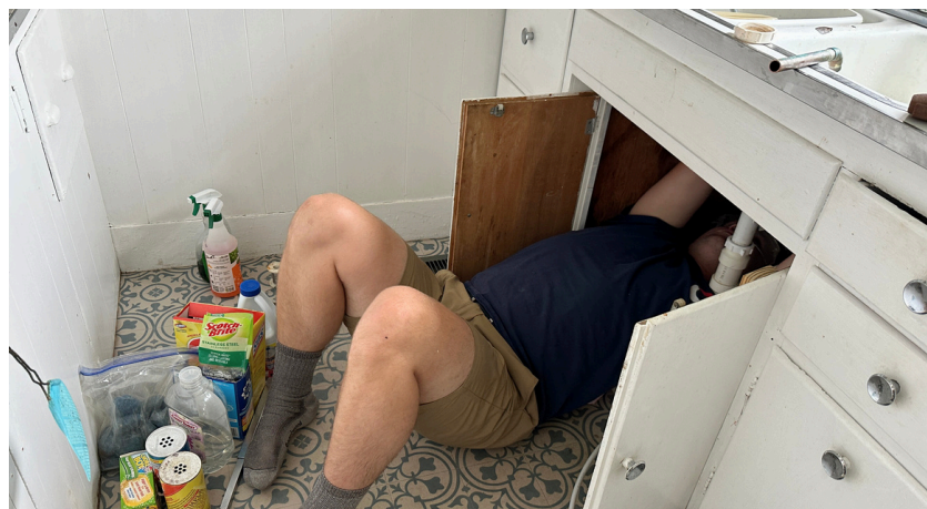
Ryan Hul repairs the Thacher Assistant Keeper House plumbing.
