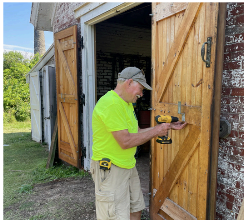
Bill Helmuth realigns the doors on the Thatcher Oil House.
