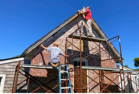
Pete Morgan and Dave Bennett paint Oil House soffit.
