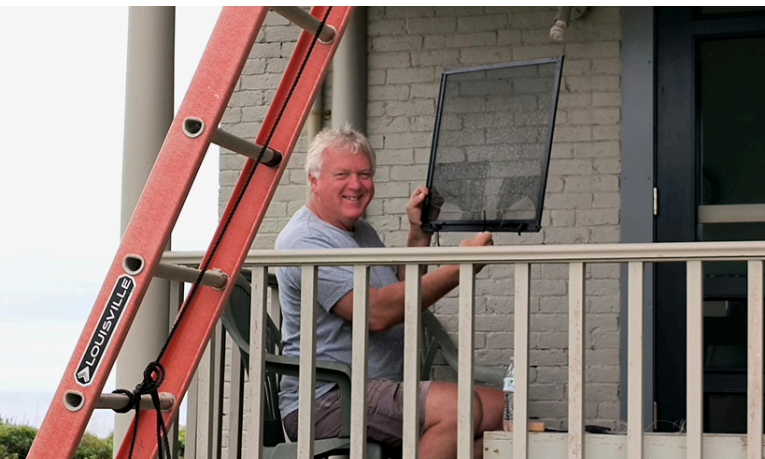
Dave Anderson repairs a screen from the Thacher Assistant Keeper House.
