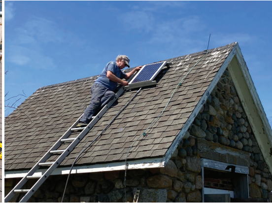
Left to right: Mike Hammerl, Meredith Glaser, and Joe Napolitano put the finishing touches on the walkway to Straitsmouth lighthouse (photo credit: Peter Bergholtz). Bill Helmuth and Peter Bergholtz complete the stairs to the Straitsmouth lighthouse walkway (photo credit: Peter Bergholtz). Norm Delisle installs a solar trickle charger for the Thatcher diesel generator battery (photo credit: Larry Haynes).
