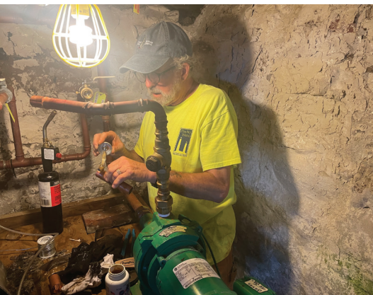
Left to right: Dave Condino replaces the water pump in the Thatcher Assistant Keeper House basement (photo credit: Norm Delisle). Dick MacPherson and Norm Delisle replace the control panel for the diesel generator (photo credit: John Fulton). Long-time keepers George & Dottie Carroll were honored with a granite bench installed in their memory on the south end of Thatcher Island.
