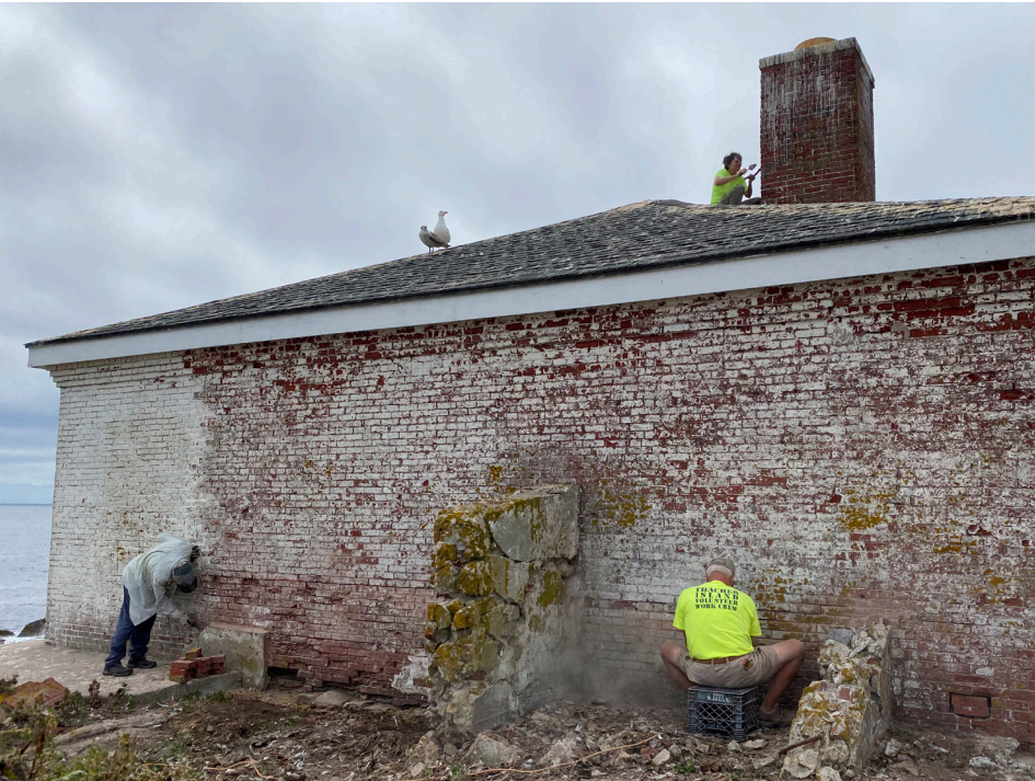
The Whistle House needed masonry repointing on a side wall and the chimney. Donna Cusick is again on the roof while Tom Mikus and Fred McGrath work from ground level.
