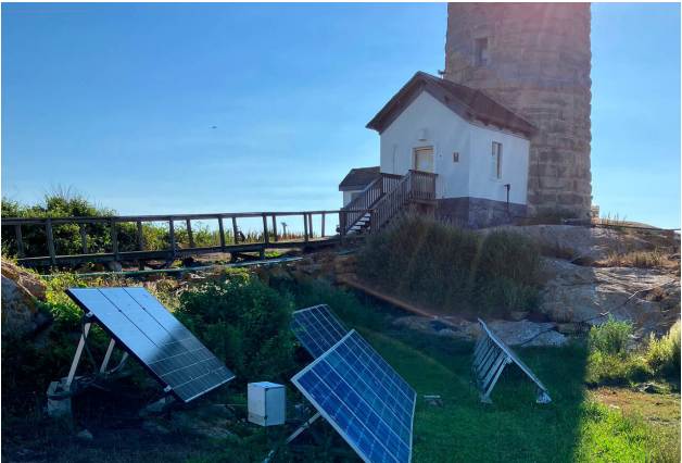
The shadow of the South Tower blocking the existing solar array
