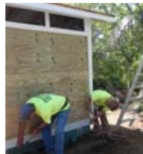
Sheathing and trim.
